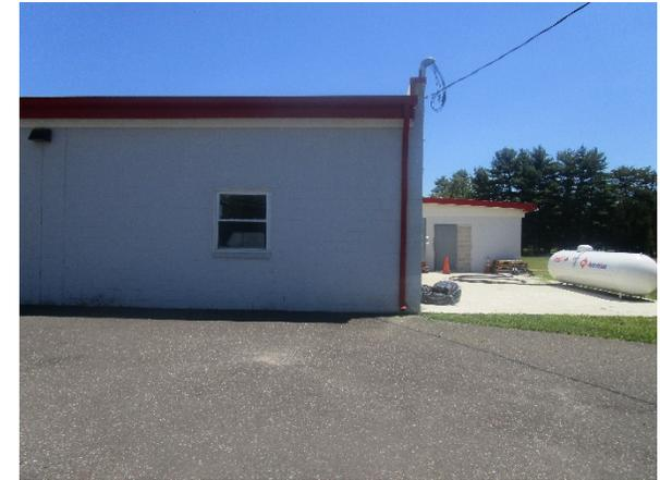
A cistern can be installed, and downspouts from the fire station's roof can be redirected into the cistern. The captured water can be used to wash fire trucks or for other non-potable uses. A preliminary soil assessment suggests that the soils have suitable drainage characteristics for green infrastructure.
