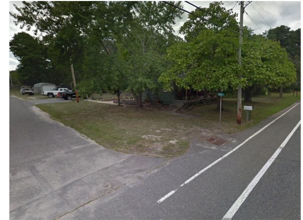
A bioretention system can be placed in the turfgrass area between Peacock Road and the house. The bioretention system will be able to capture runoff from the road by bypassing the catch basin. A preliminary soil assessment suggests that the soils have suitable drainage characteristics for green infrastructure.
