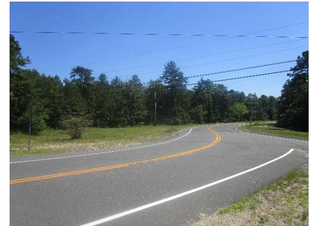
A bioswale can be installed along the roadside to capture runoff from the road. Bioswales are landscape features that convey stormwater from one location to another while removing pollutants and allowing infiltration. A preliminary soil assessment suggests that the soils have suitable drainage characteristics for green infrastructure.
